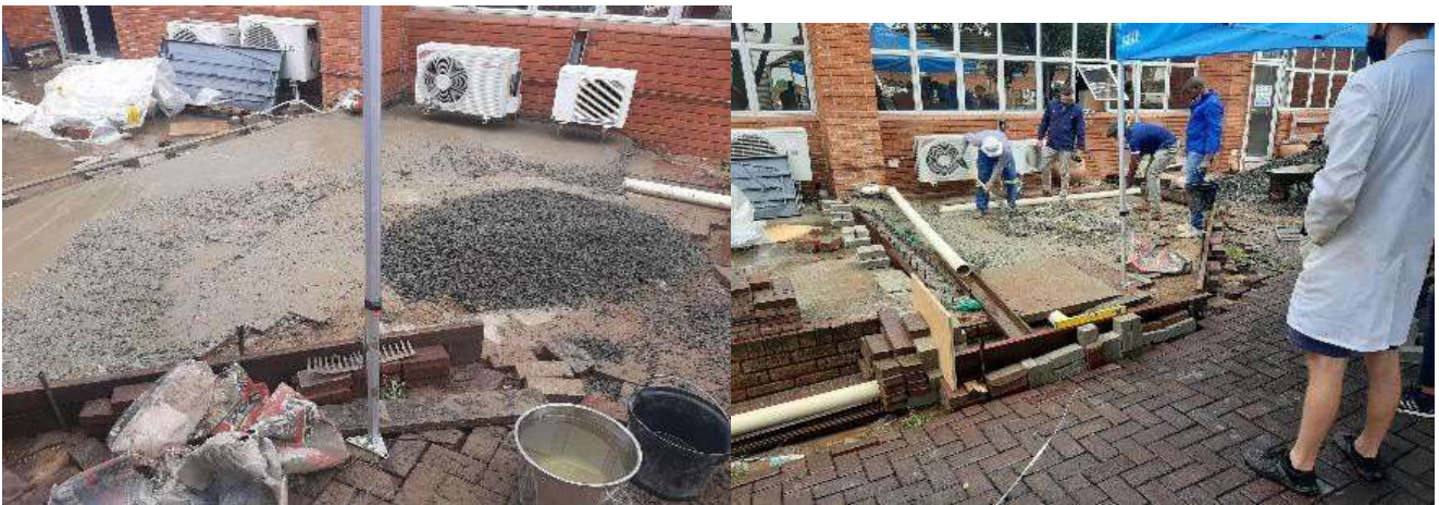
Figure 7 - Addition of testing area (built by students)
