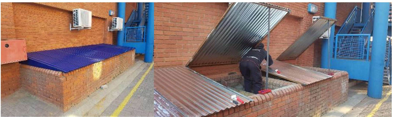
Figure 9 - Aggregate storage bins
