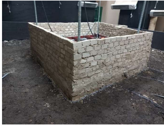
Figure 3.18: Completed SM house
